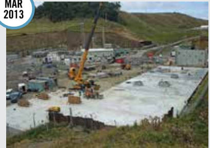
Foundations installed and MCC walls erected
