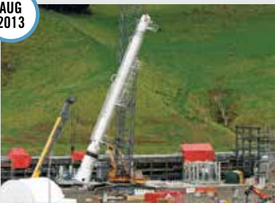
Stabiliser column installation
