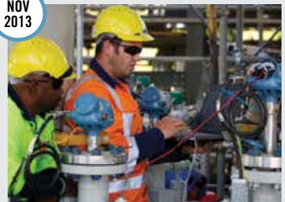
Pre-commissioning activities underway
