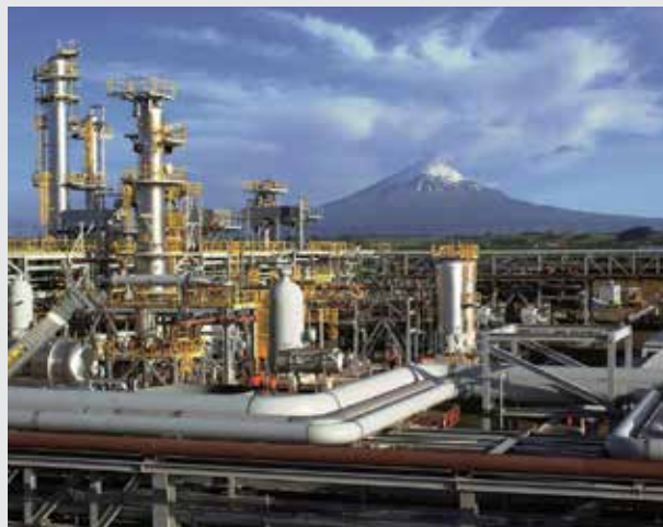
Gas from the offshore Kupe field is piped to the onshore production station (above).
