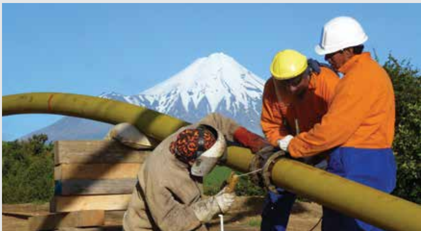
Energyworkers constructing new pipeline with minimal negative environmental impact.
